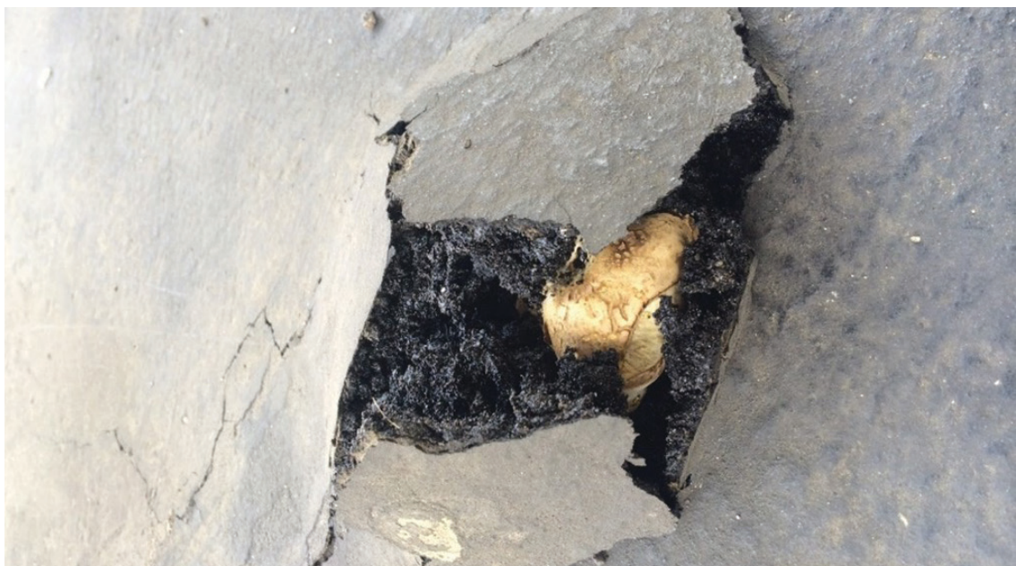
■ Figure 1. A fungus (likely from the genus Pisolithus ) generating enough force to crack solid asphalt (reprinted courtesy of Frank McDonough).
