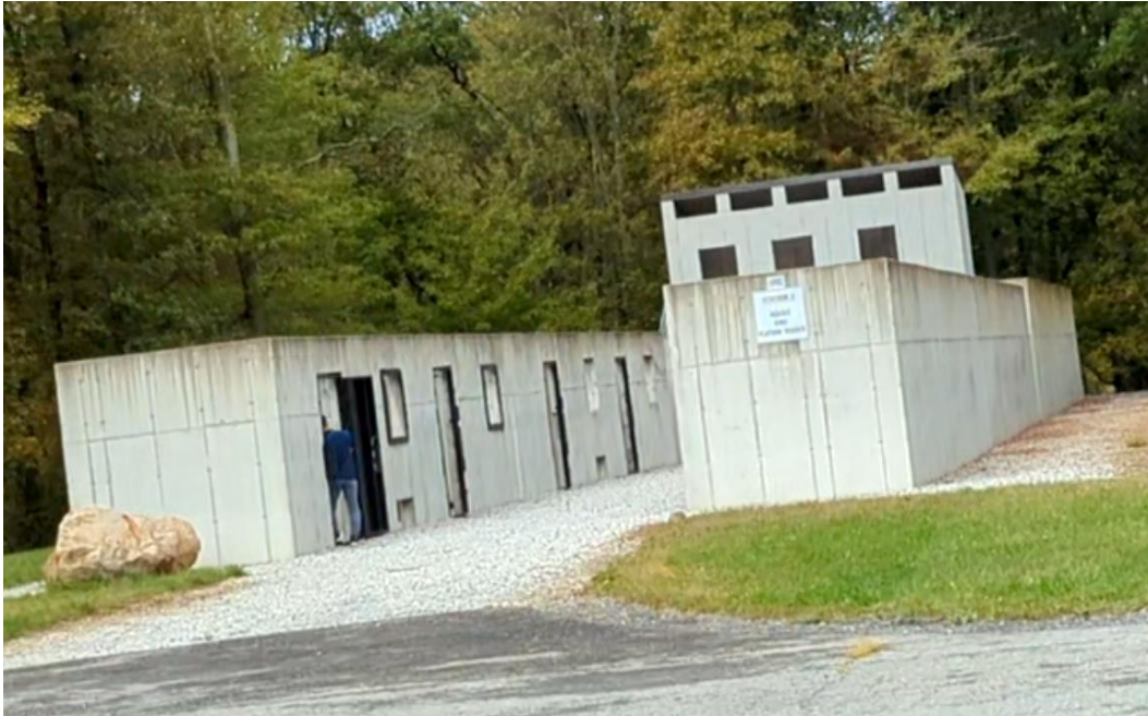
Figure B-4. Station 2 concrete rooms for room clearing.
