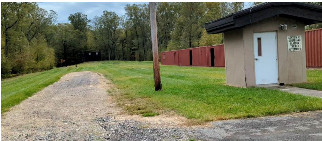
Figure B-3. Station 2 CONEX boxes and cleared area.
