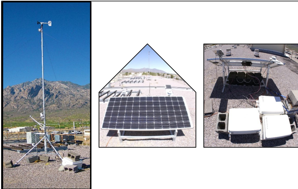
Figure 1. AIHPA Testbed (MMT and PT systems).
