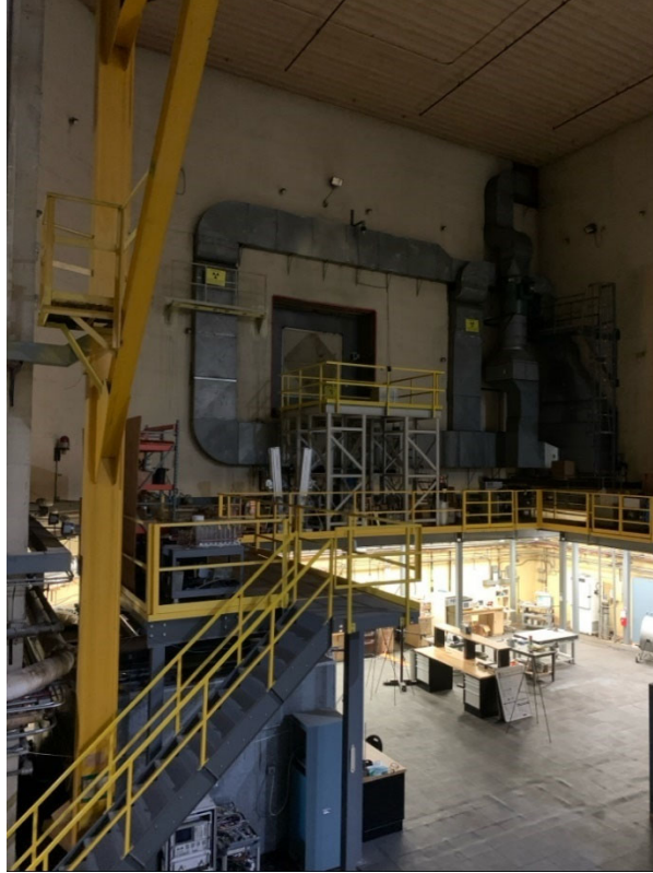
Figure 7. Inside the High Bay looking in the direction of the Bay Wall. Legacy radiation-warning signs can be seen on the position of ducts in the High Bay corresponding to the position of the passthroughs seen in Figure 6. The Dimple Plate is seen in the rectangular recess. Since the removal of Aurora in 1996, the High Bay has been adapted to use for a variety of projects, including construction of a mezzanine (gray flooring surrounded by yellow railing) and, on top of that, a platform just in front of the Dimple Plate. The mezzanine is used only for storage, and the platform is only used to monitor radiation levels on the High Bay side of the Dimple Plate. The better-lit area below the mezzanine is used by personnel on a routine basis for work on unrelated projects.
