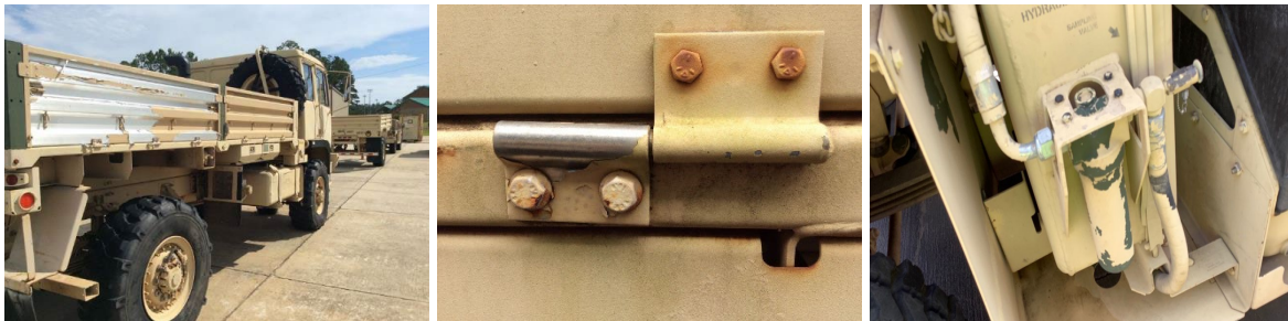
Figure 20. Examples of delamination (cargo bed side, hinge, hydraulic line).
