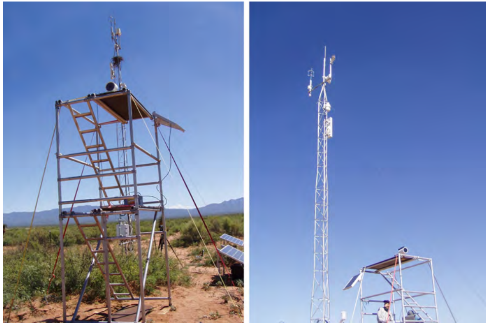
Fig. 4 Phase 1 BLS 450 setup at MSA towers; BLS transmitter at Tower 1 (left) and BLS receiver at Tower 2 (right)
